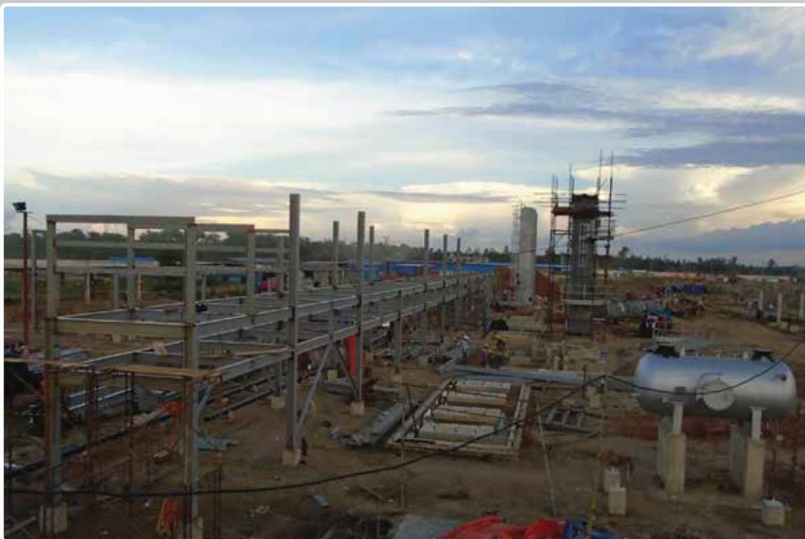
Equipment, Vessel, Piperack Installation.
